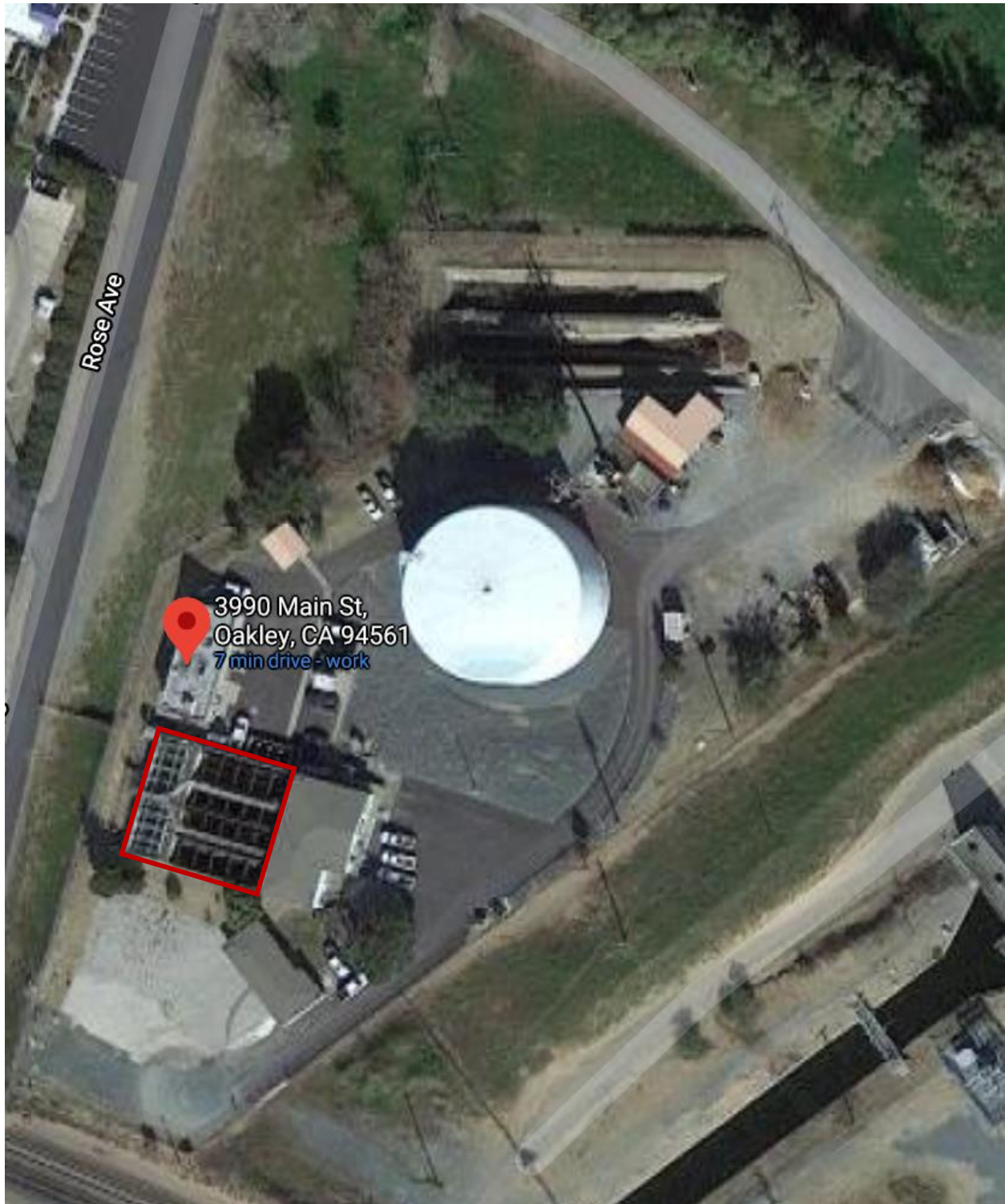
Ground mount or possible installation on top of old clarifiers (red outline).
