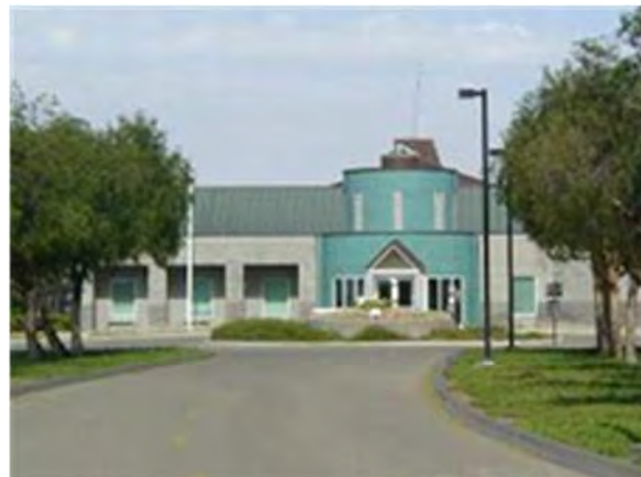
The Randall-Bold Water Treatment Plant is one example of a shared facility within the East Contra Costa County Region
