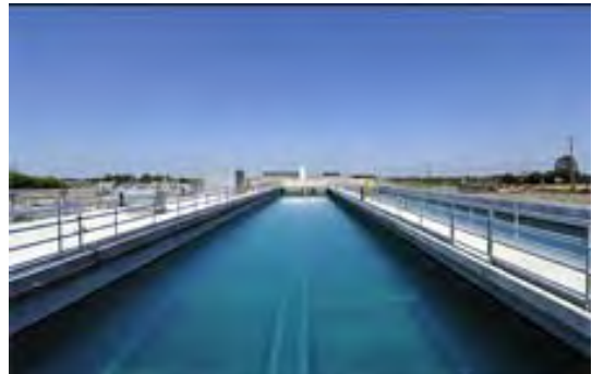
City of Brentwood Water Treatment Plant.
