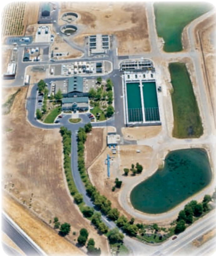
Randall-Bold Water Treatment Plant
