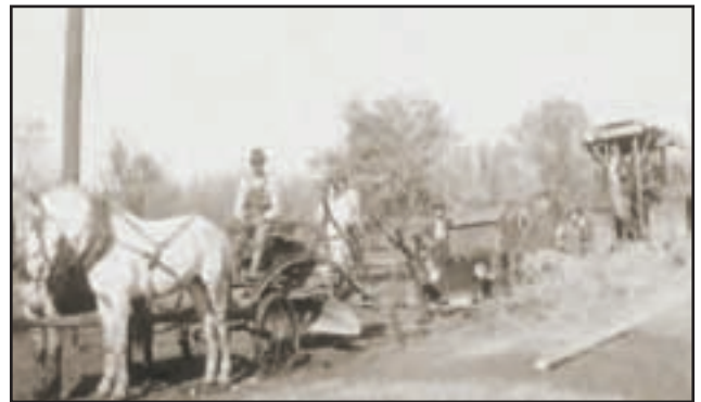
Water has always been critical to our community's development and economy. Here, Ernest and Ruth Crockett are paving Live Oak A venue around the turn of the 20th century using water from their own well.
