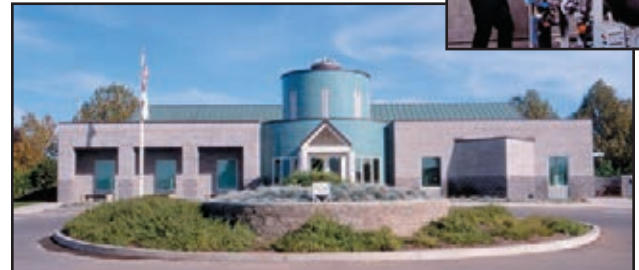
Your water is treated at the Randall-Bold Water Treatment Plant, which is jointly owned by Diablo Water District and Contra Costa Water District.
